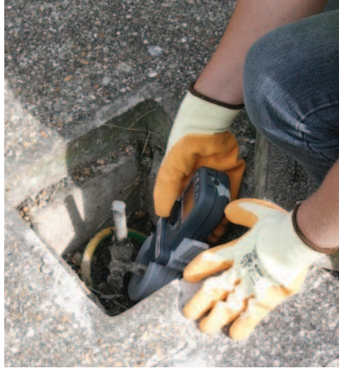
The DET14C is shown measuring a ground spike in a ground well.
